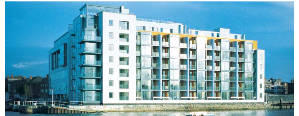
Southbank Quay, Grand Canal Dock, Dublin 4.
